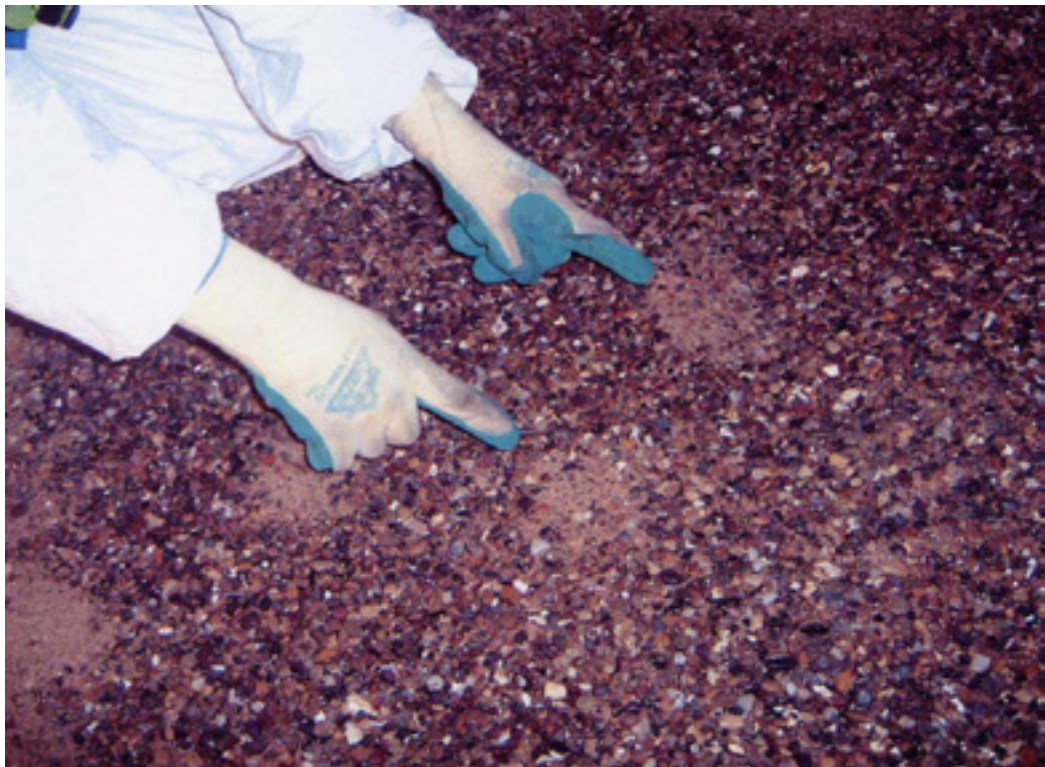
Figure 13: Filter B, jetting through gravel and sand migration
