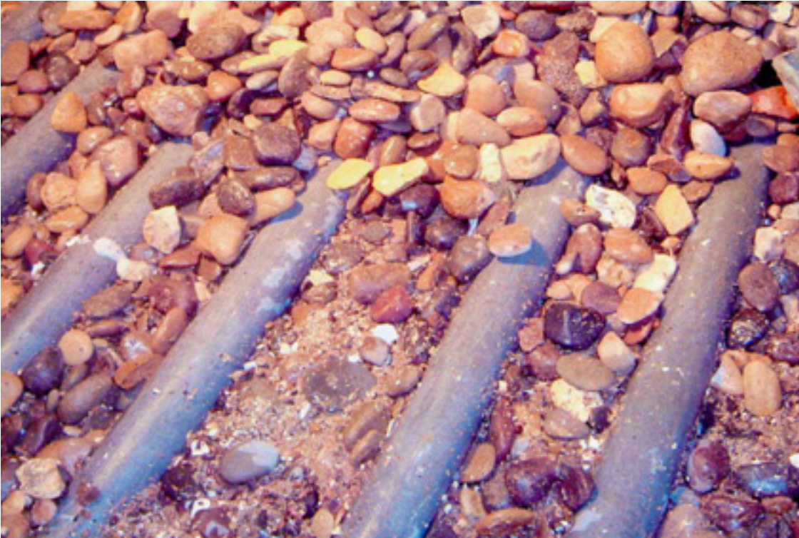
Figure 11: Filter A, Large amount of fine sand, silt and seashell fragments between laterals.
