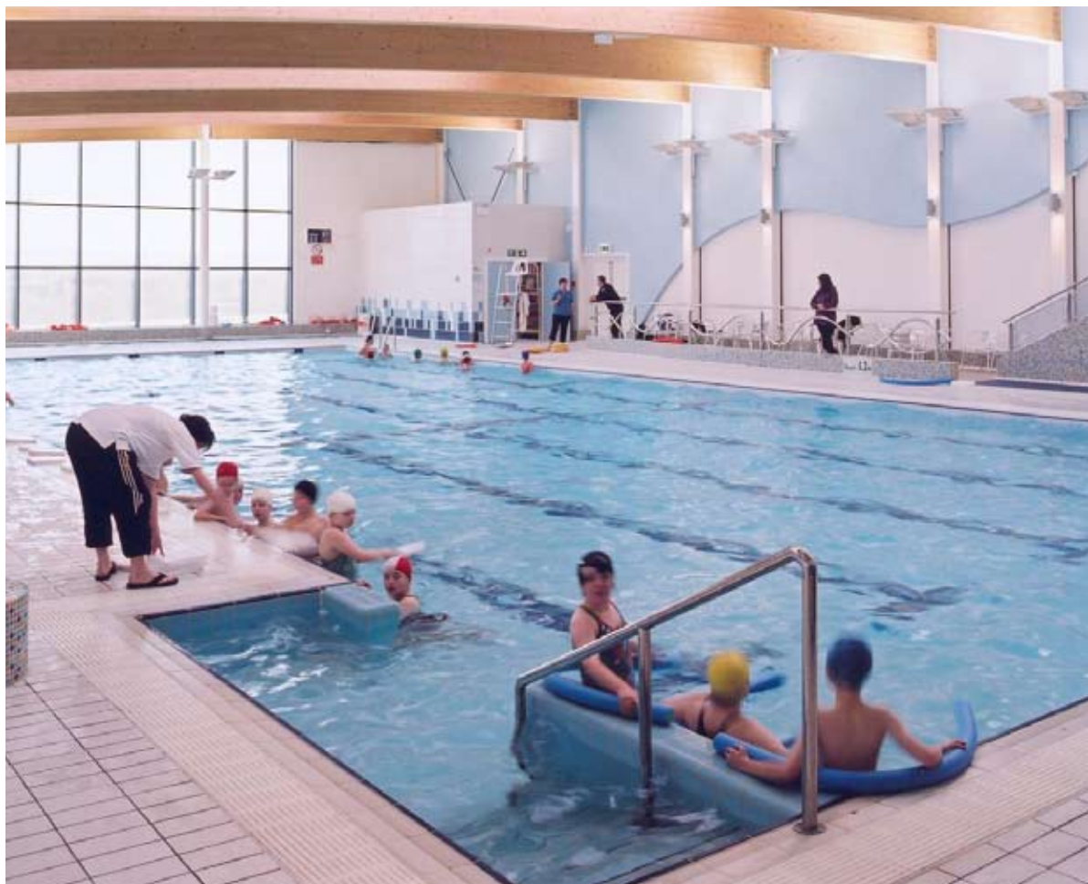
Recessed 'easy going' steps allow easy access to and from the water for all users
