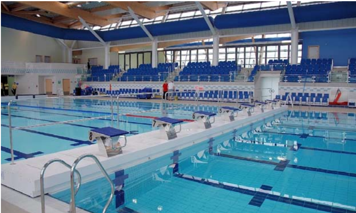
The bulkhead allows divided simultaneous use of two areas of a single swimming pool
