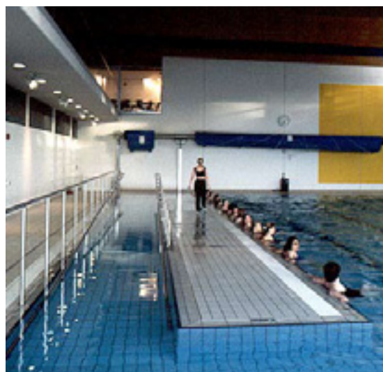
Ramp access and projecting platform adjacent to a teaching area in a specialist pool
