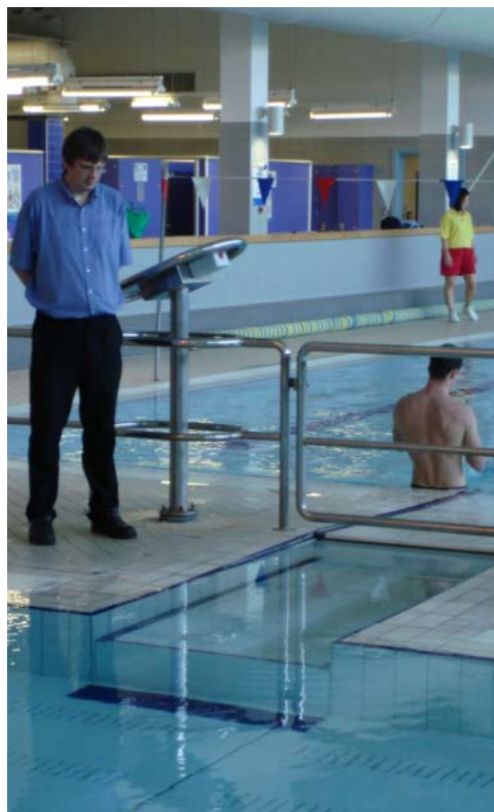
A submersible pool surround lift integrated into the pool as part of the pool surround can provide a dignified access to the pool for wheelchair users
