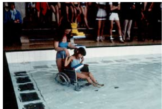
Movable floors allow a wide variety of uses
