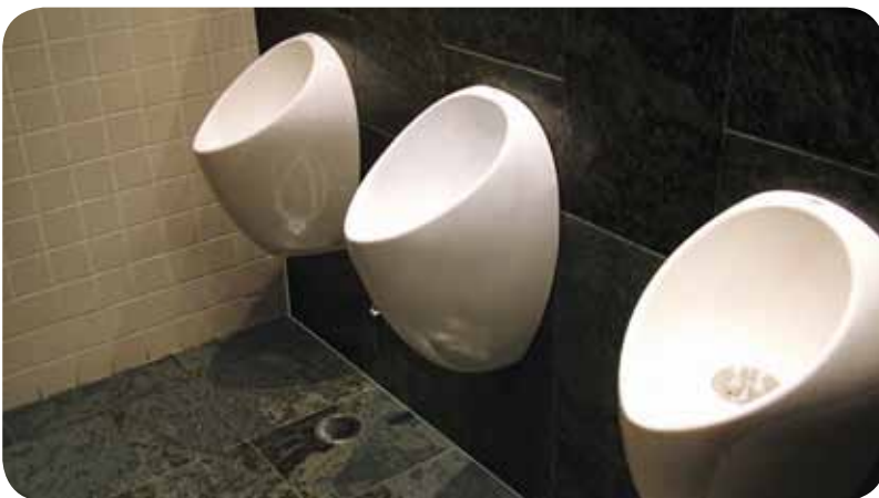
Replace or retrofit conventional urinals with low-flow urinals and regularly maintain and adjust flush valves and sensors
