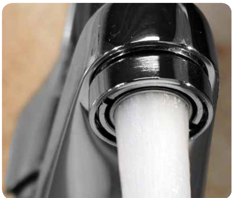
Install vandal proof housings over basin tap flow restrictors to prevent theft
