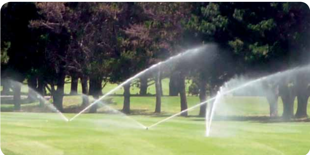
Inspect irrigation systems regularly to make sure sprinkler heads and timers are working properly
