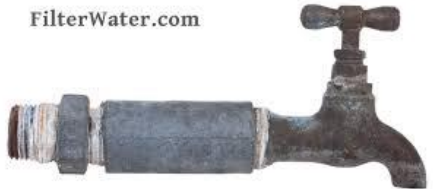
Lead pipes found in older homes
