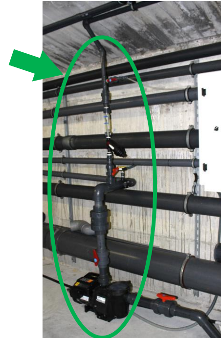
Recirculation pump for disinfection and pH neutralisation
